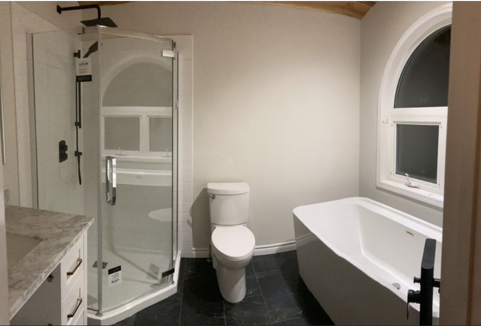
Bathroom plumbing and fixtures
