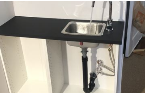
Sink and faucet installation
